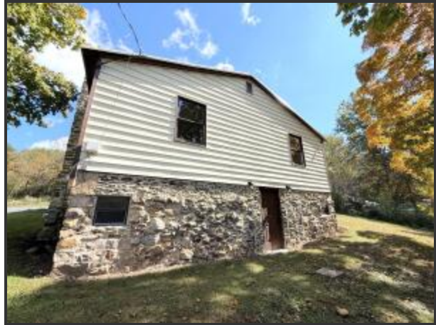
Side with door to basement/crawlspace
