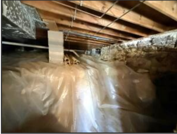
Crawlspace with 6 mil vapor barrier
