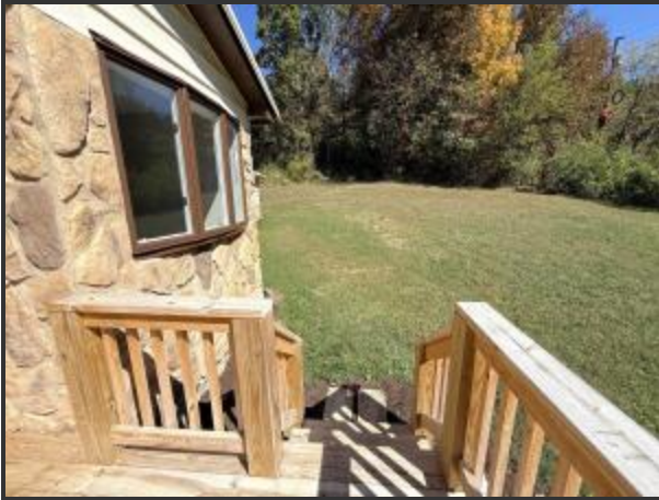
Steps from rear deck to back yard
