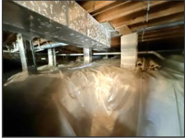
Crawlspace with 6 mil vapor barrier
