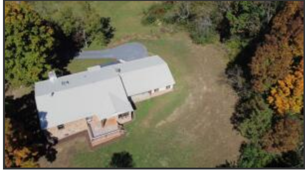
Aerial from rear
