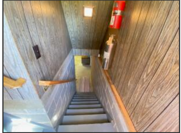
Stairs to lower level
