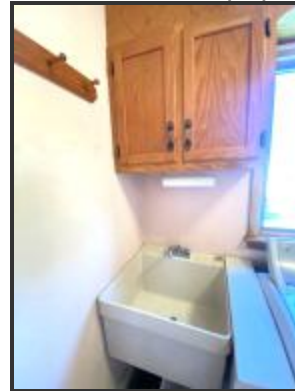
Laundry Room wash sink
