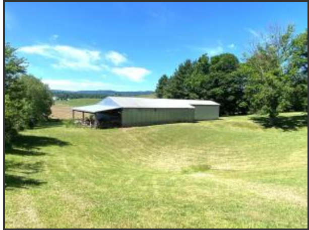
Side/rear view of storage building
