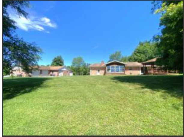
View from rear towards house and storage building
