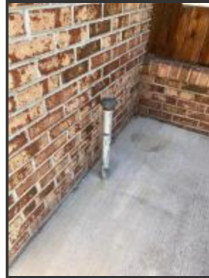
Fuel oil pipe at back door
