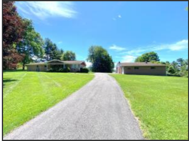
Entry from Denmar Rd
