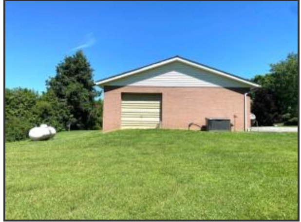
Side garage/workshop. Generator and propane tank.
