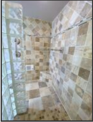
Primary Bathroom walk-in shower with built-in bench and electric heater
