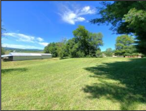
Side view of storage building
